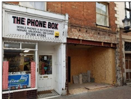
Photograph 7: Unit under alteration at 8 High Street
