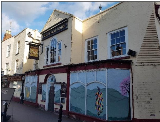
Photograph 6: Vacant former Talbot Head Hotel
