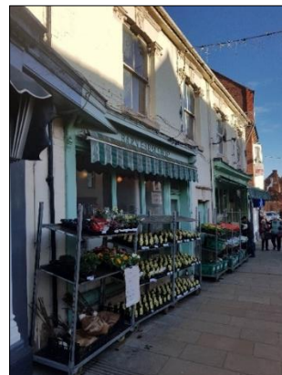
Photograph 5: Shopfront along Market Street
