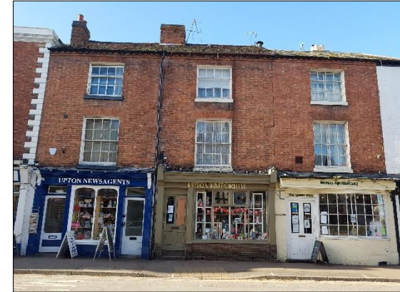
Photograph 3: Shop frontages along Old Street
