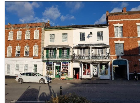
Photograph 5: View of 1-3 High Street
