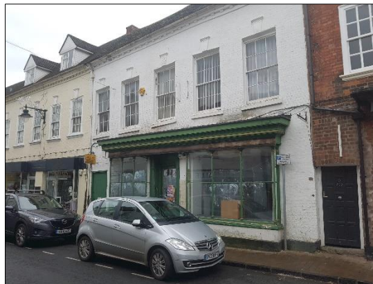
Photograph 9: Vacant unit on High Street
