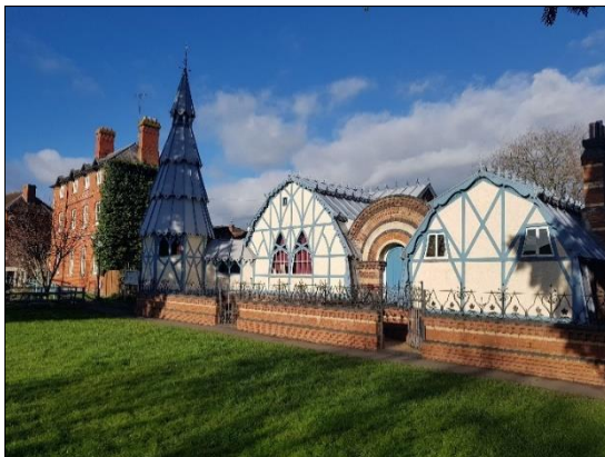
Photograph 4: Tenbury Wells Pump Rooms
