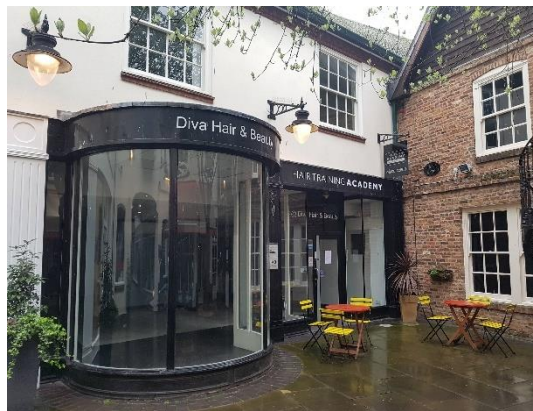
Photograph 8: Vacant unit at Reindeer Court
